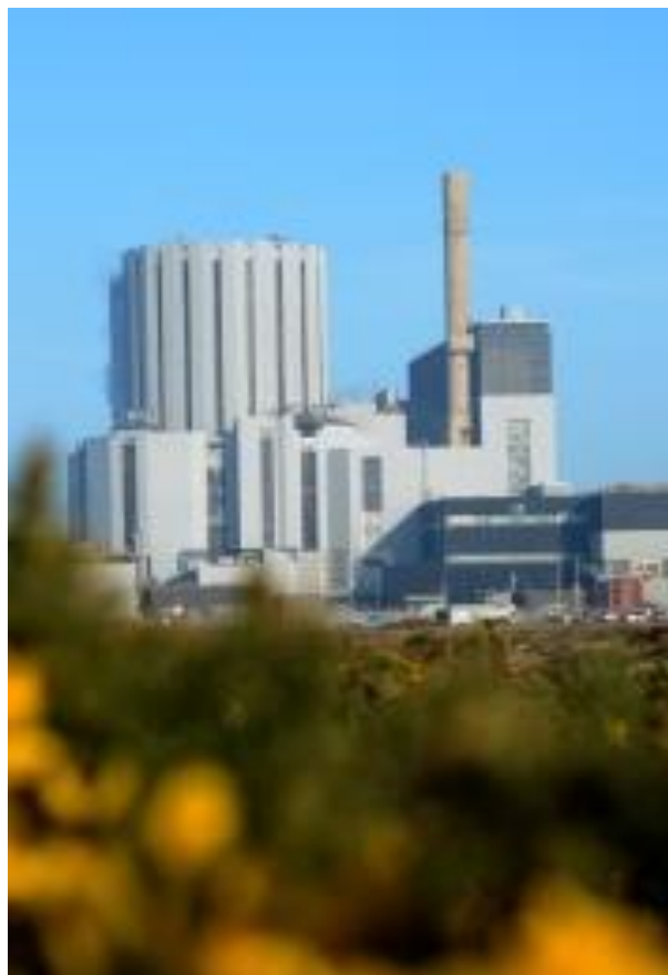
Dungeness Power Station – one of our workplaces
